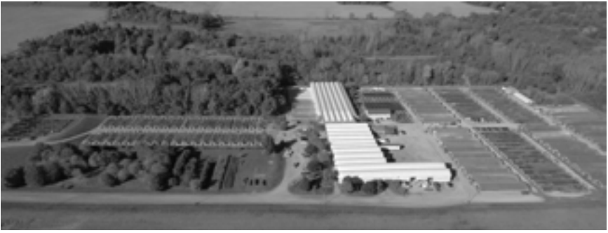
Above: Shawnee North, Main Farm, Office, and Loading Dock (24 acres)
